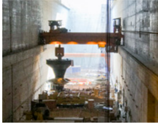
The oil-free Kaplan runners for Xayaburi are the largest and most powerful built to date.
