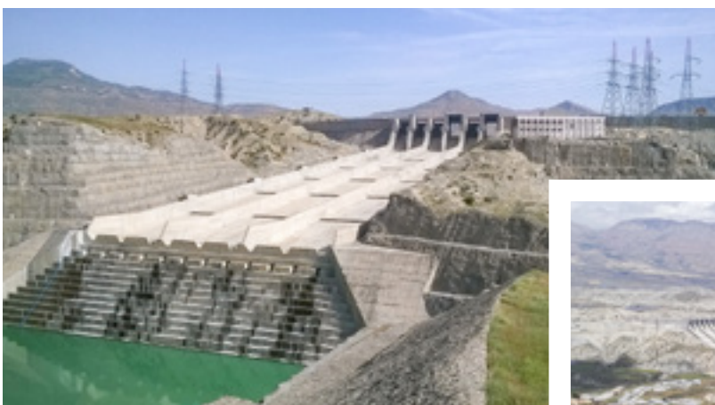
With six powerful and top modern generation units and a total output of 1,224 MW, Ilisu will significantly increase the power supply in southeastern Turkey.
