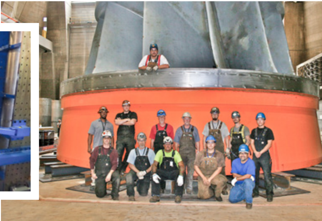
The scope for the upgrading contract comprises the complete dismantling of the turbine and the generator units, inspection of all components and refurbishment and reassembly of the units on-site.
