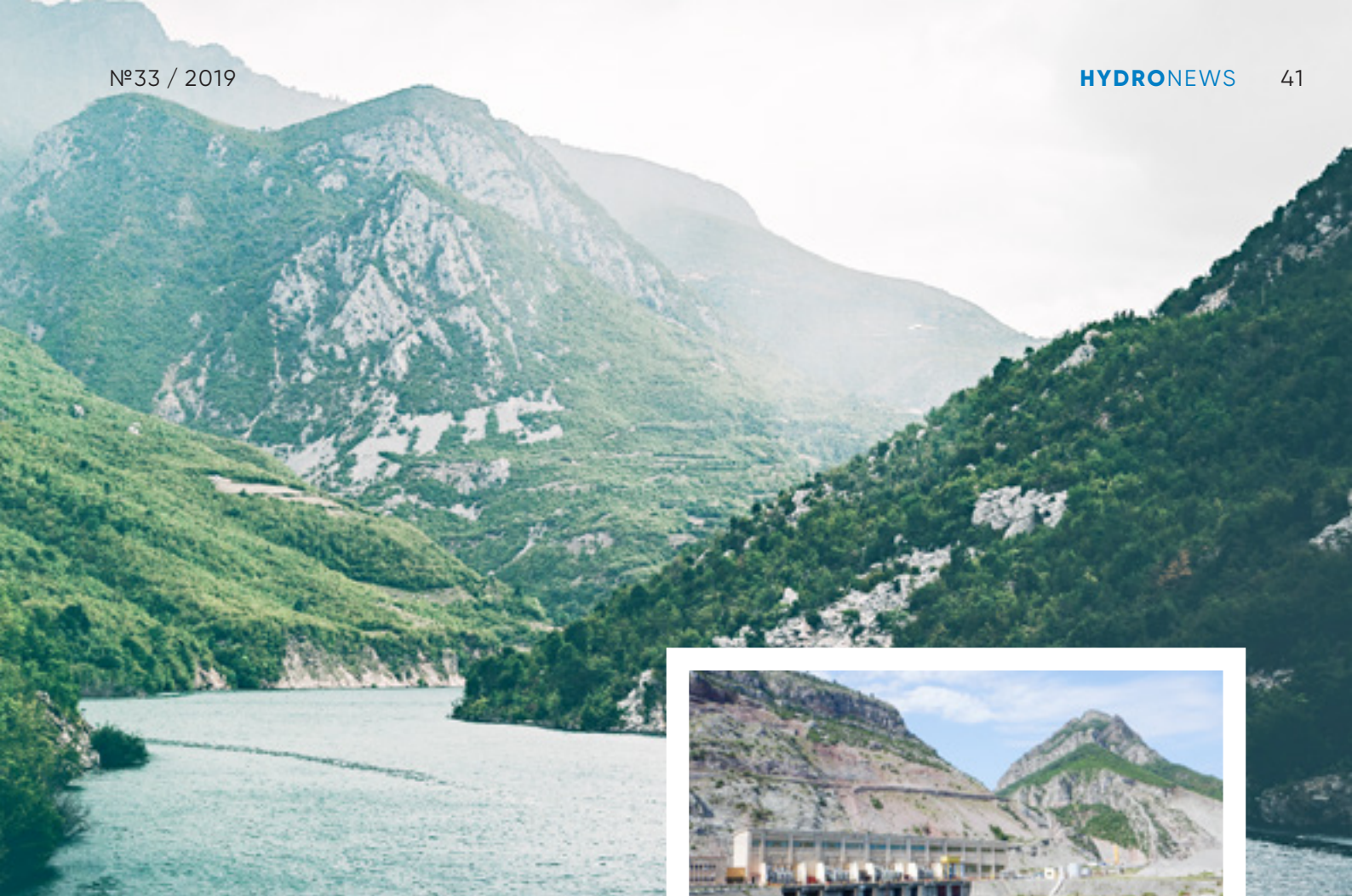
With 600 MW, Komani is the largest hydropower plant in Albania, producing more than 30% of the country's total electricity demand.
