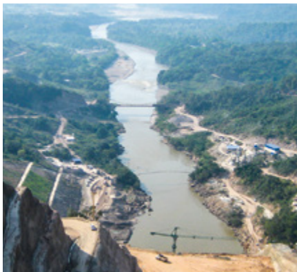
Aerial view construction site and river
