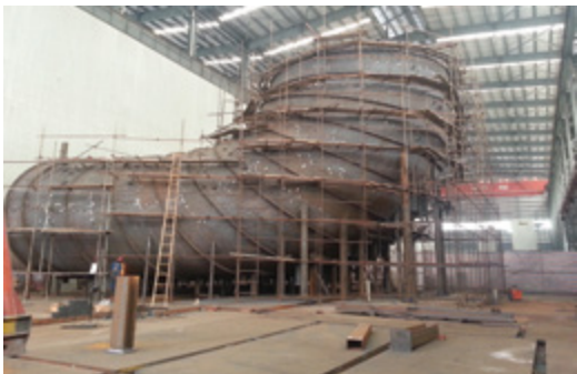
Draft tube installation
