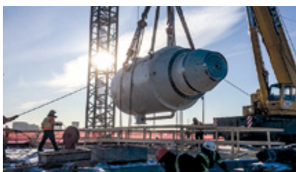
Installation of Bulb turbine
