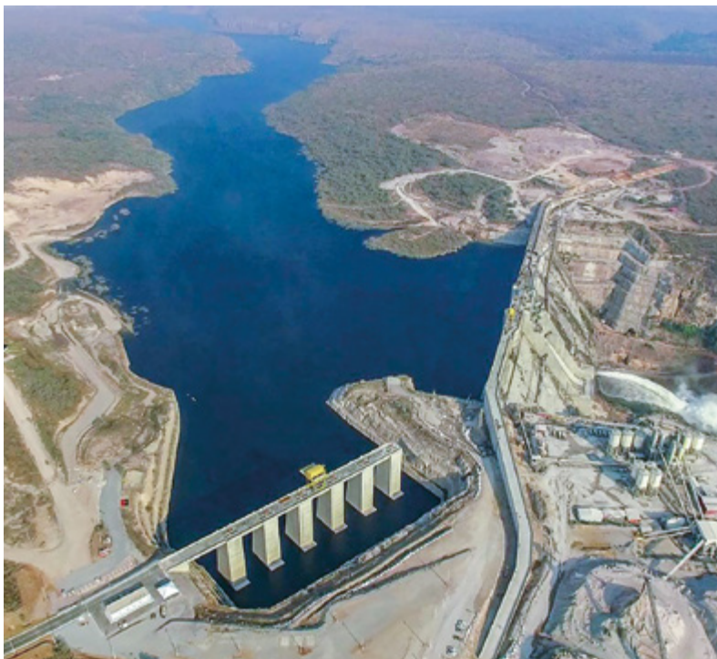
View of powerhouse, dam and area
