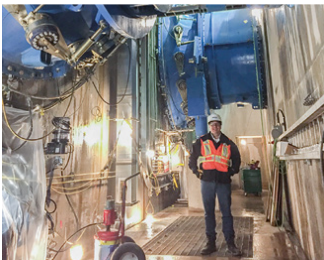
Installed Bulb turbine
