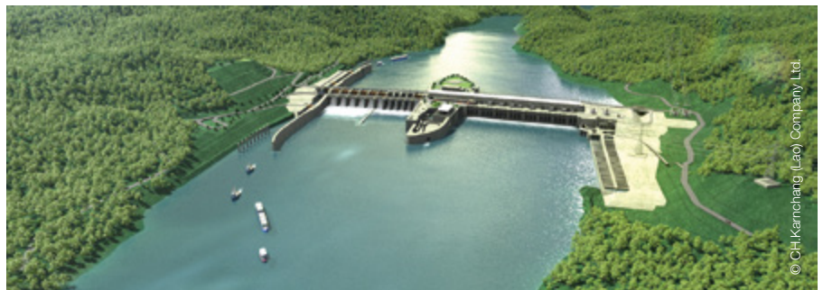
Navigation lock, spillway, intermediate block, powerhouse and fish ladder
